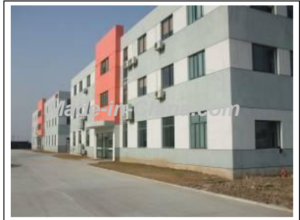
Description: Workshop building
